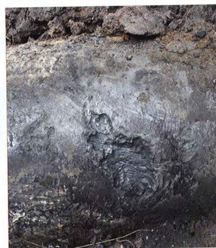
Mechanical removal of graphitised zone in a corroded cast iron pipe.
